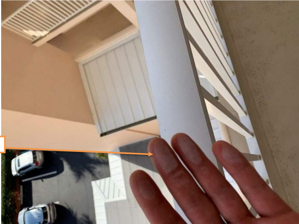
Figure 34: 5 th floor walkway.
