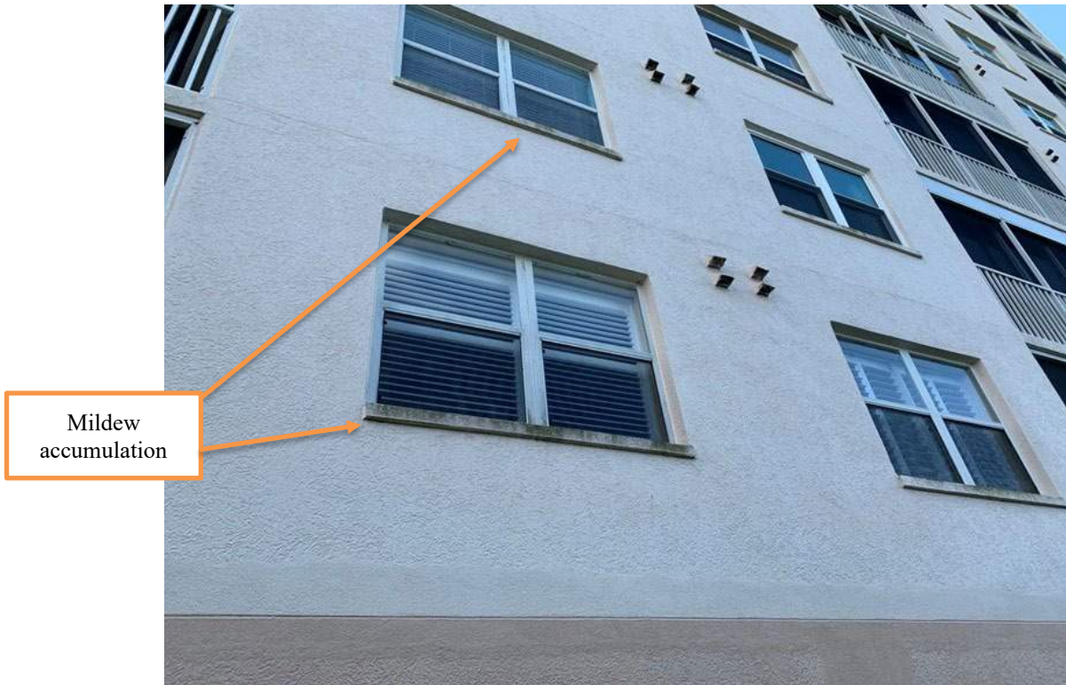
Figure 12: North side exterior, ground floor
