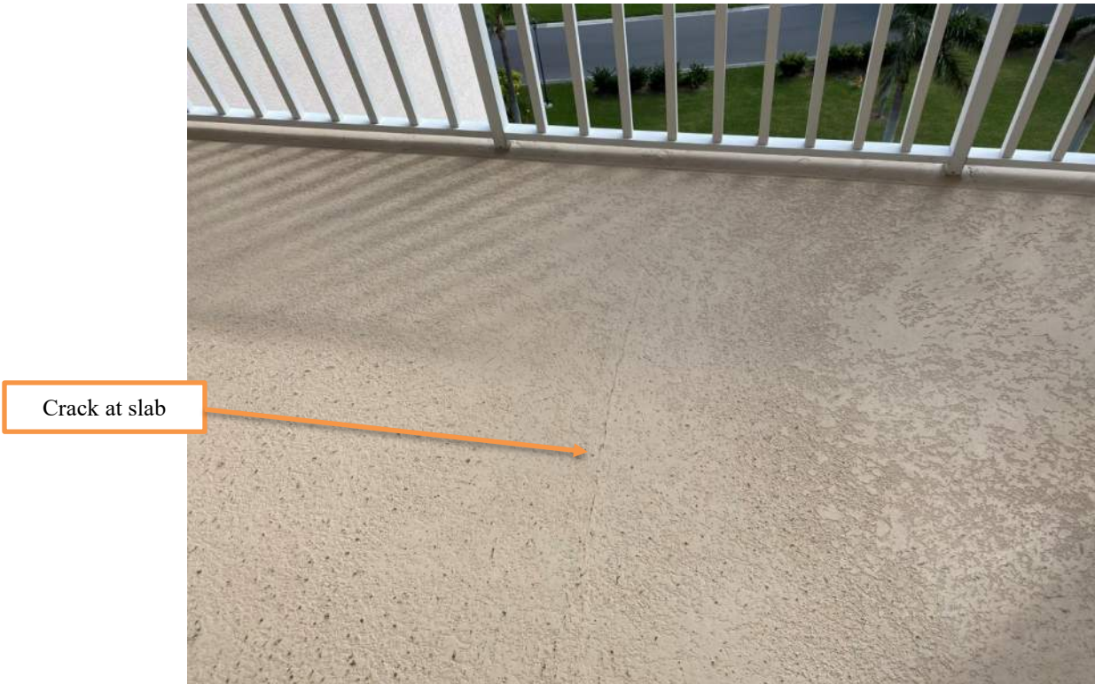
Figure 8: 8 th Floor Walkway
