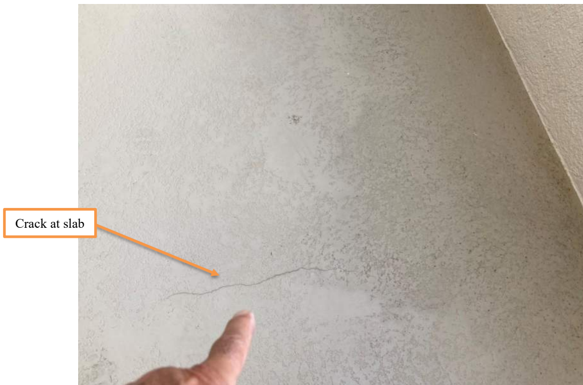
Figure 7: 2 nd Floor Walkway.
