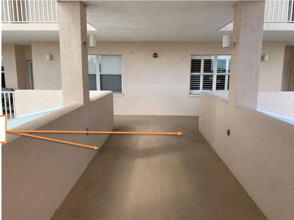
Figure 28: 2 nd floor walkway.
