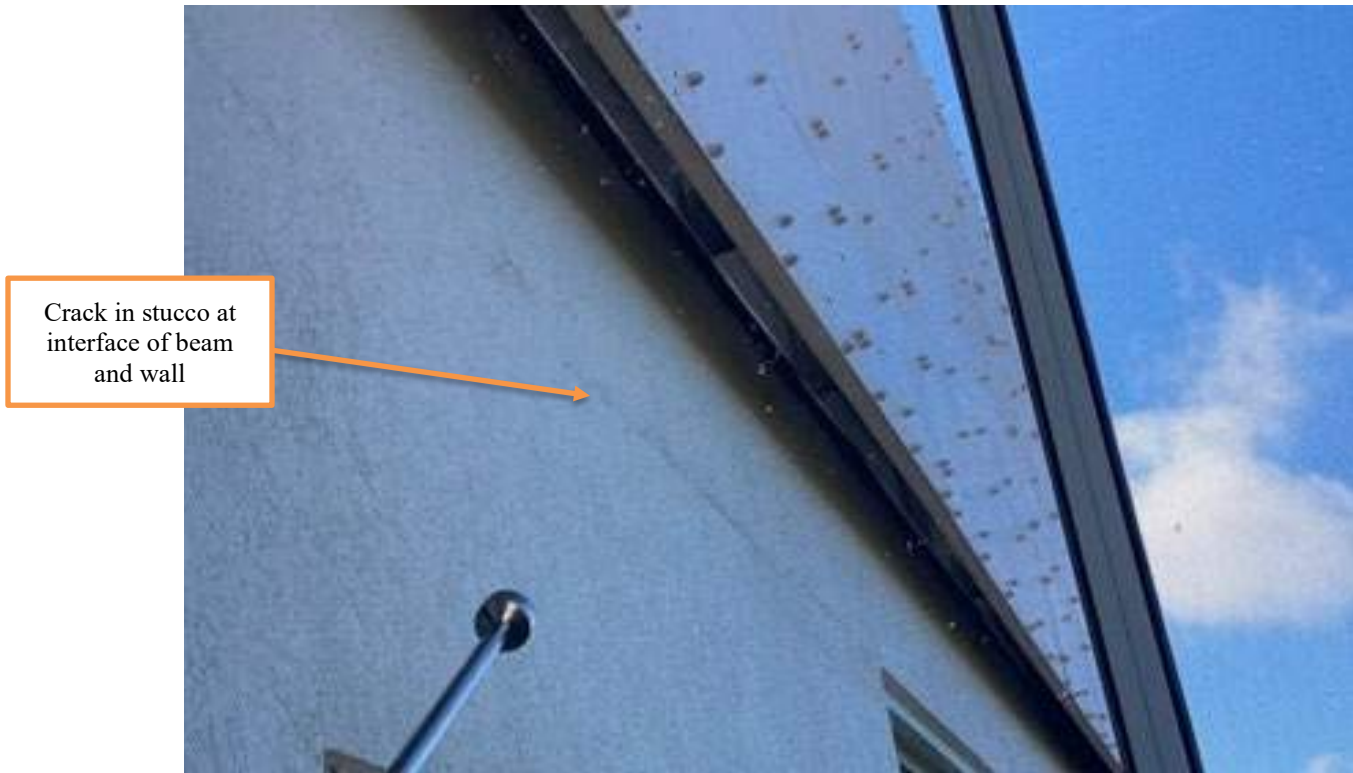
Figure 10: View of exterior wall from Unit 802 balcony.
